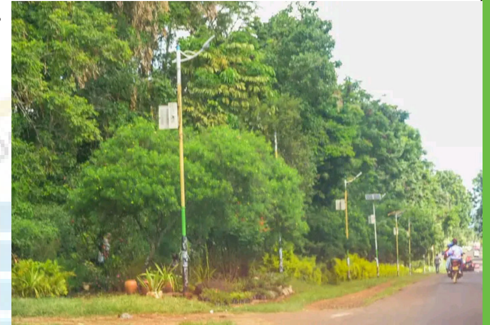
STREET LIGHTS ALONG EMBU - MERU HIGHWAY
