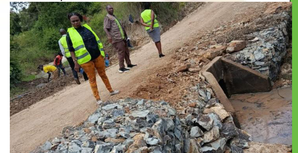
CULVERT INSTALLATION ENSURIG SAFER LOADS
