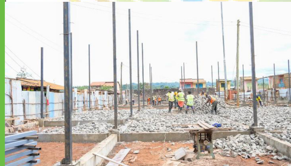
SITE CONSTRUCTION OF MODERN MARKET IN EMBU.
