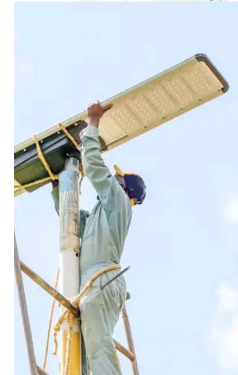
INSTALLATION ON PROGRESS
